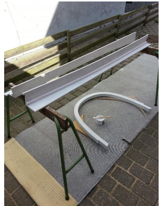
Final paint on wooden parts
